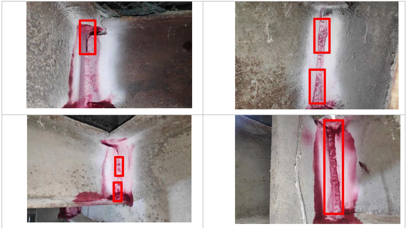
Figure 7. Dye penetrant inspection (beam and column structure)
